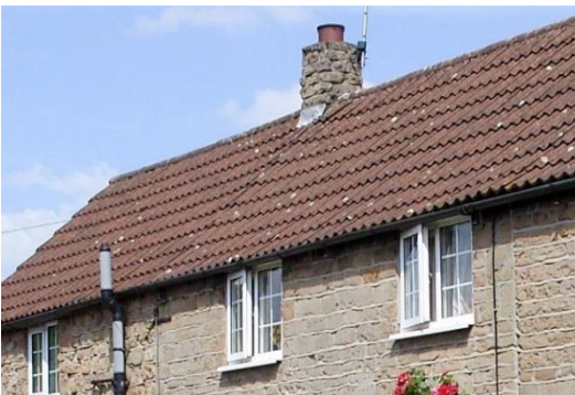
Photo – casement windows
