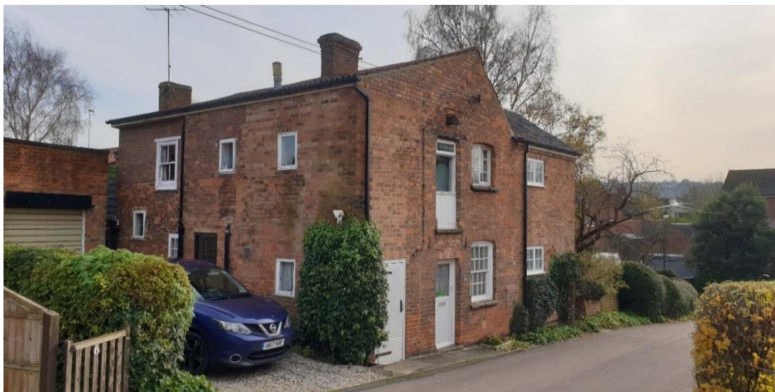
Photo 29: No 45 Main Street
