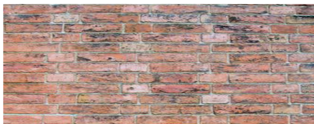
Photo of Flemish Bond type brickwork
