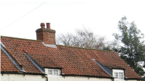
Photo raked dormers at Church Street, Lambley
