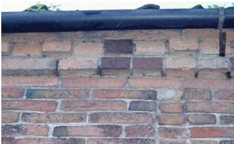
Photo 57: Irregular Flemish Bond with Dog-toothed eaves.
