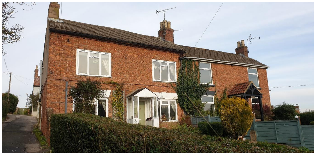
Photo 53: Cottages on Chapel Lane
