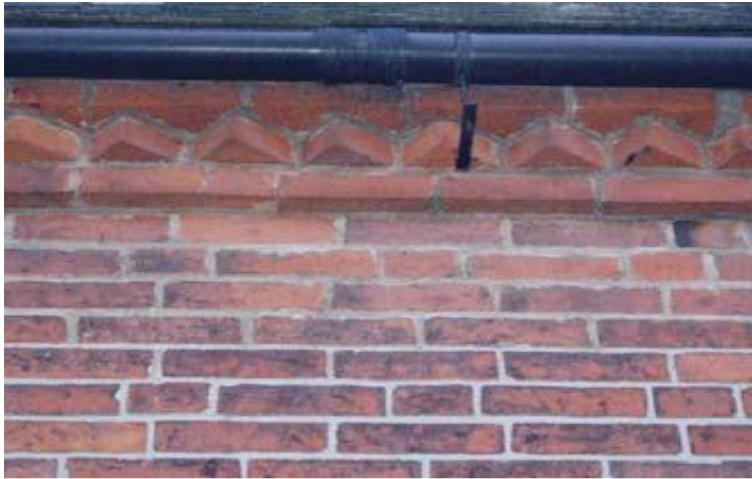
Photo 57: Irregular Flemish Bond with Dog-toothed eaves.
