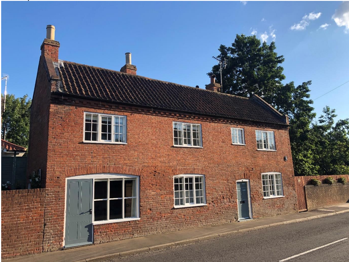
Photo 28: No 18 Main Street
